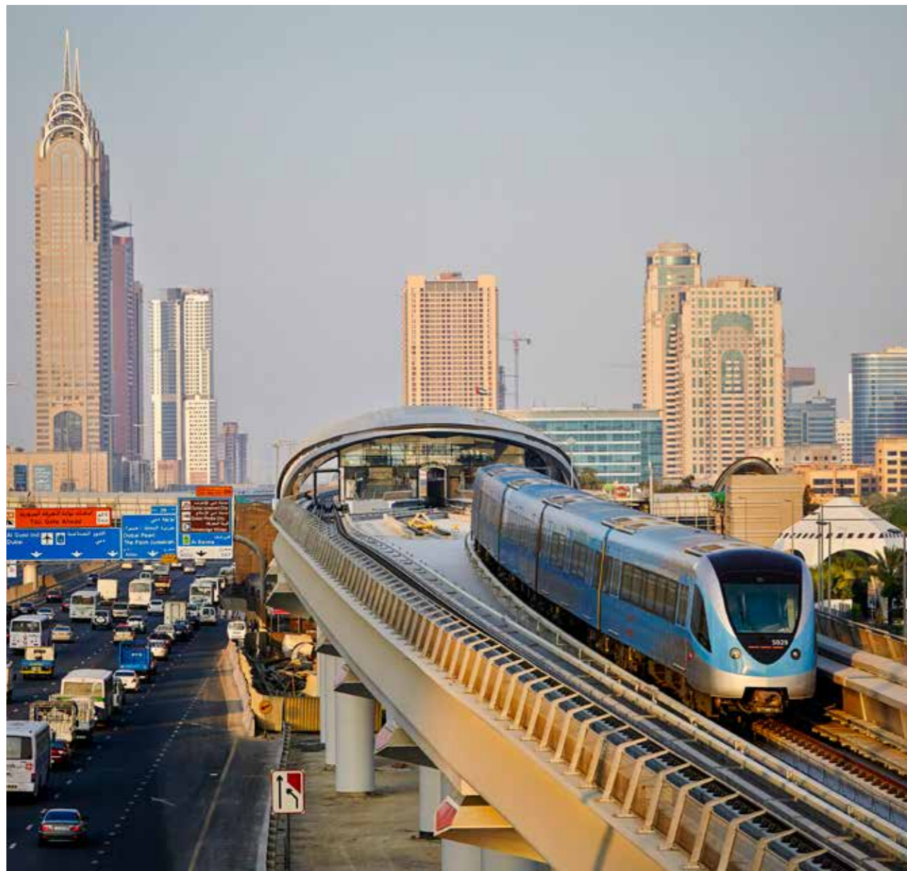
The Dubai Metro is the world's longest fully automated metro network in the world.
